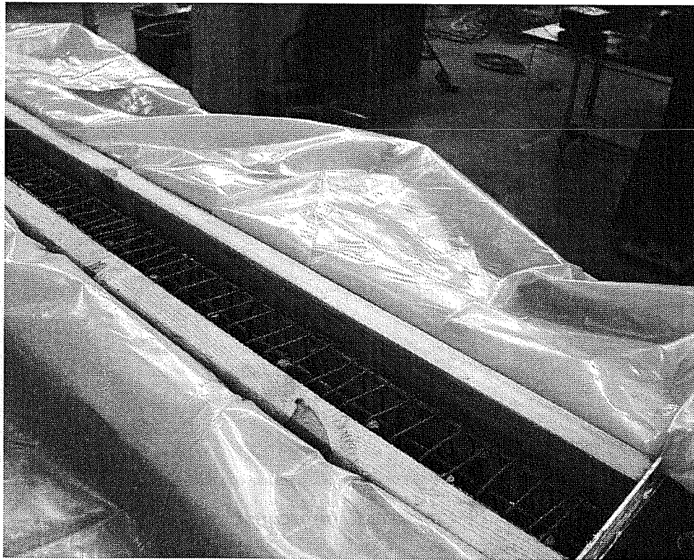
Figure 5.40 Concrete Stiffener Formwork
